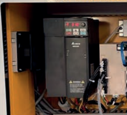
High-performance 15HP inverter
